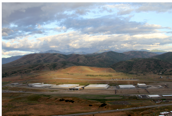
Figure 3.1 – NSA Utah Data Center, Source: Parker Higgins [21]
